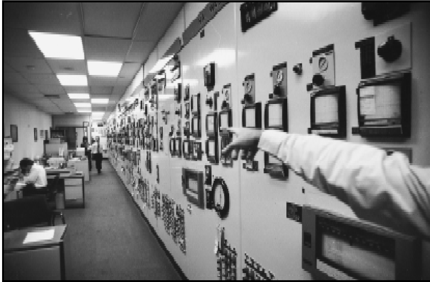
F Canyon Control Room. From this room, operators controlled the processing of irradiated reactor targets. The targets were dissolved in acid so that plutonium could be separated from the uranium and highly radioactive fission product wastes. F Area, Savannah River Site, South Carolina. January 6, 1994.
