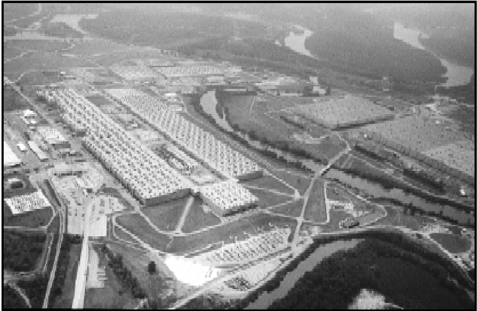
The K-25 Gaseous Diffusion Plant enriched uranium for nuclear weapons and commercial reactor fuel from 1945 until 1967. When first built, the U-shaped K-25 building was one of the largest roofed structures in the world, covering nearly 43 acres. K-25 Gaseous Diffusion Plant, Oak Ridge, Tennessee. June 12, 1962.
